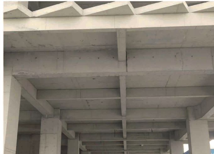
Demoulding effect of roof and beam formwork
