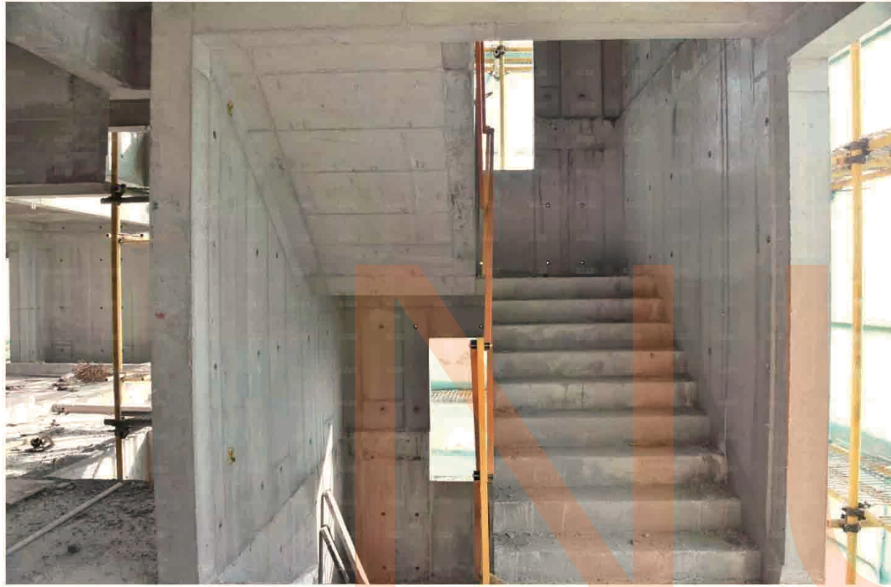
Demoulding effect of ladder formwork
