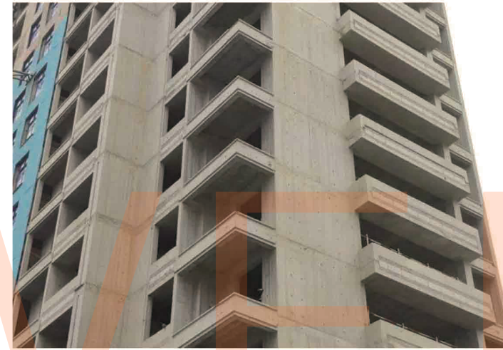
Exterior wall formwork demoulding effect
