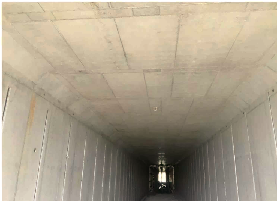
Tunnel formwork demoulding effect
